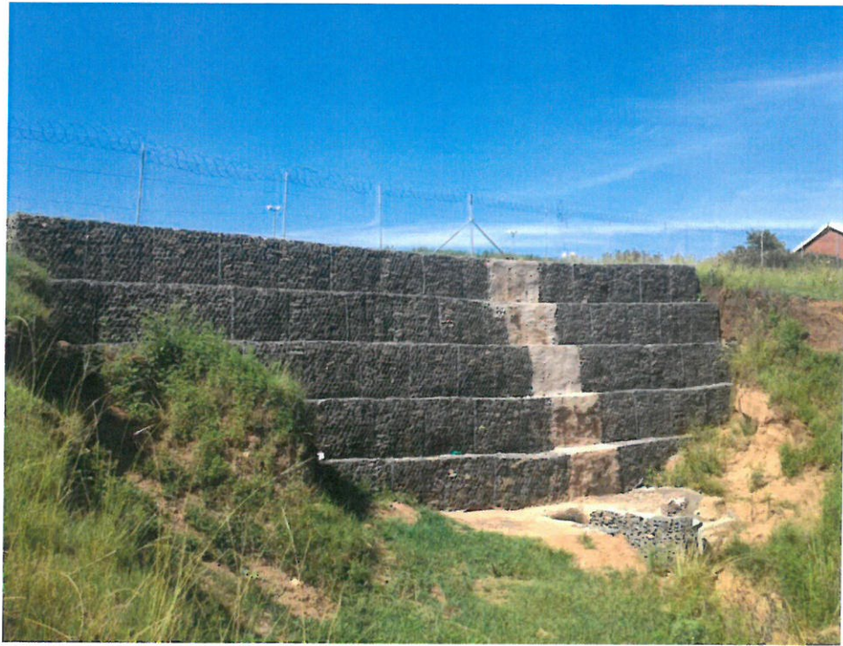
Gabion installation at Ficksburg WWTW
